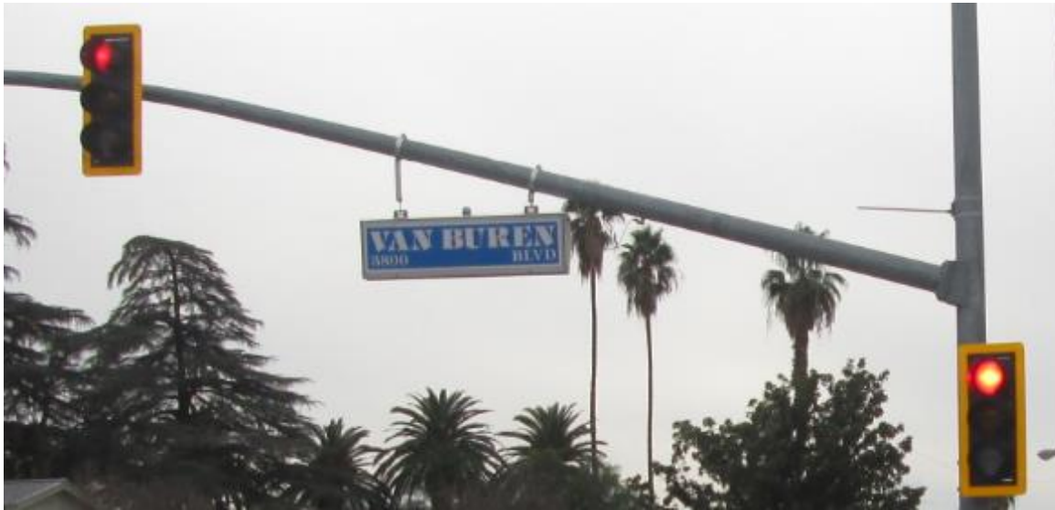
Retroreflective yellow borders installed at Magnolia Avenue at Van Buren Boulevard
