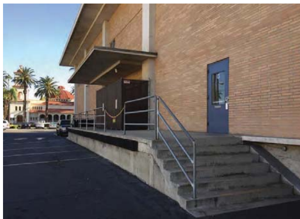
Existing loading dock with bumpers, stairs and canopy.
