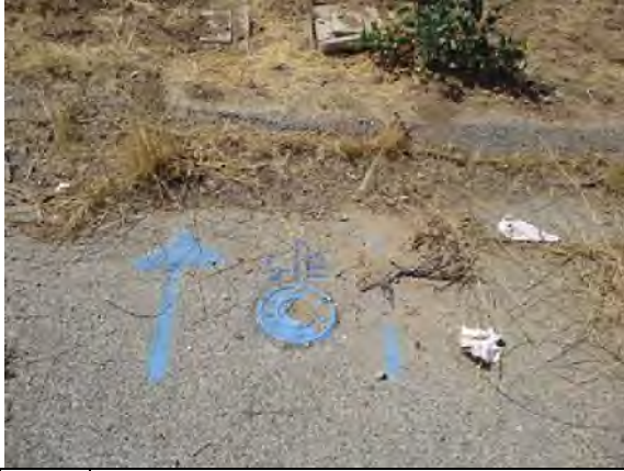
Photo #25: Water line markout
