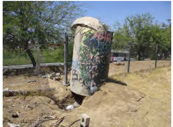
Photo #22: Apparent broken sewer pipe (on end) at south portion of property
