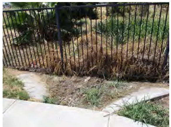
Photo #6: Concrete swales for drainage onto Sonic Ct
