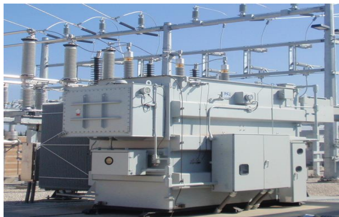
Typical Substation Power Transformer
