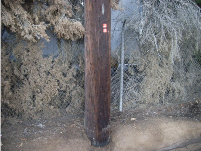
POLE TAGGED FOR REPLACEMENT
