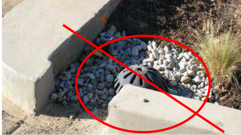
Figure 6: Incorrect Placement of an Overflow Inlet.
