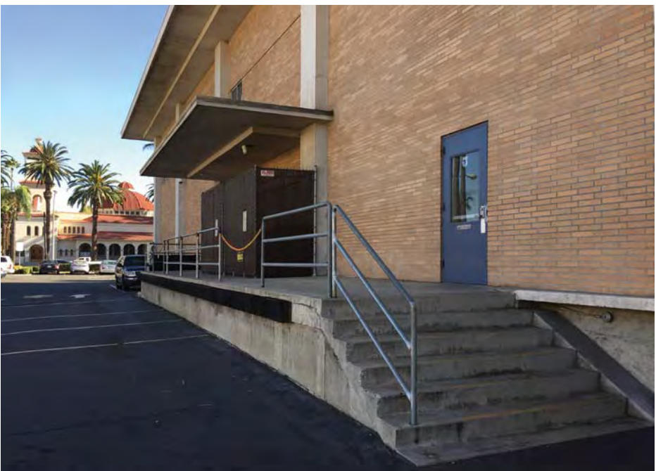
Existing loading dock with bumpers, stairs and canopy.
