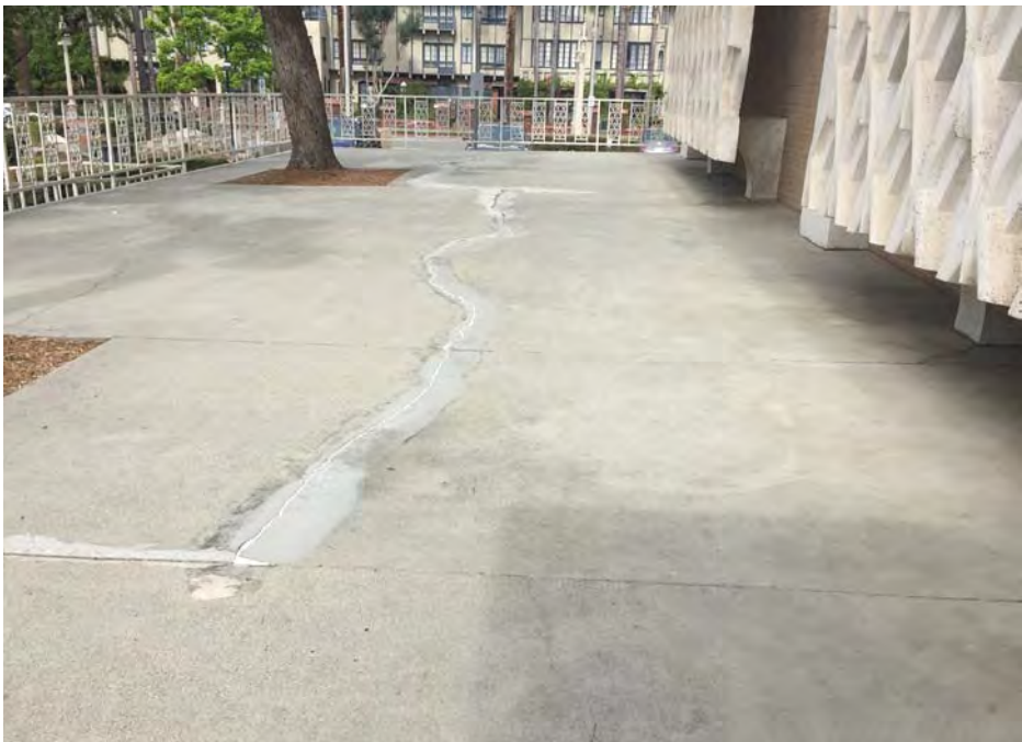
Concrete at podium, in poor condition, will be replaced.
