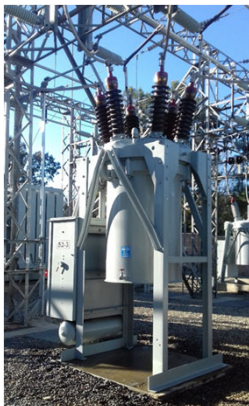
Typical Oil Circuit Breaker (Aged Unit)
