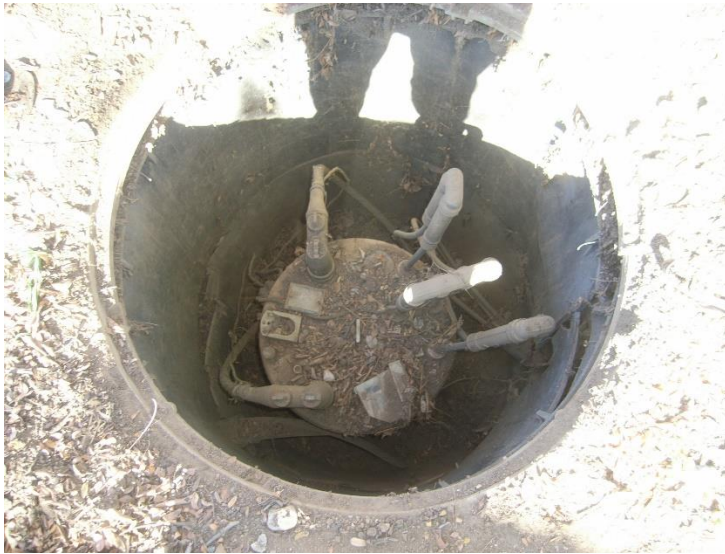
Deteriorated Buried Transformer Enclosure
