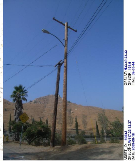
Double “Buddy” Pole to be removed
