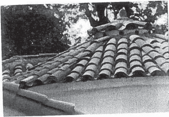
Photograph above shows Two-Piece Red-Clay Barrel Mission Tile at 4648 Ladera Lane. Below is historic one-piece "S" Mission Tile located at 4651 Ladera Lane.
