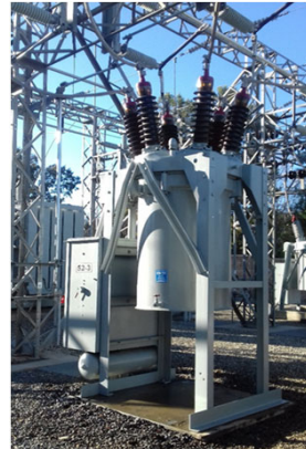
Typical Oil Circuit Breaker (Aged Unit)
