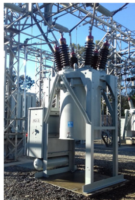
Typical Oil Circuit Breaker (Aged Unit)
