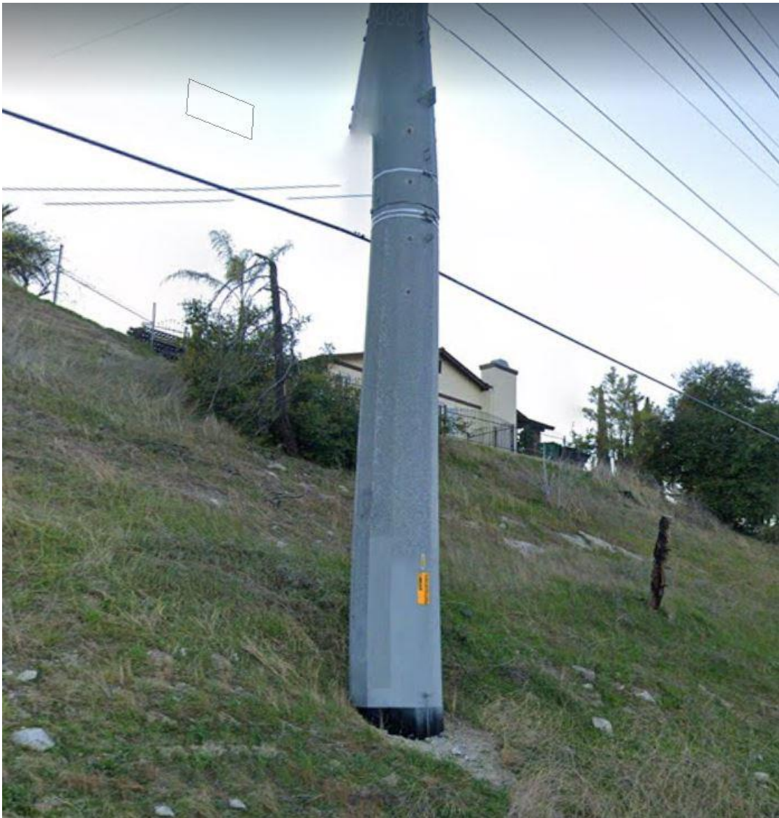
Typical steel pole base directly embedded into the ground
