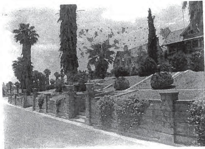
*Public improvements along Indian Hill Road installed in 1906. Improvements include faux-granite retaining walls, cement plant urns, sidewalks, raincross street-light fixtures, concrete bollards and iron chain.*
