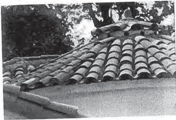
*Photograph above shows Two-Piece Red-Clay Barrel Mission Tile at 4648 Ladera Lane. Below is historic one-piece "S" Mission Tile located at 4651 Ladera Lane.*
