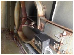
AHU-3 Supply Housing Access Door: The supply air housing access door is not sealed and is leaking supply air. This should be sealed to achieve maximum system performance.
