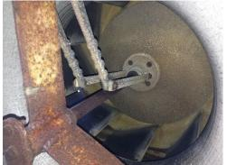
AHU-2 Chilled Water Coil: The chilled water coil condensation water pan is rusty and corroded.
