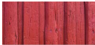
1 THIN STARTLING RED CEDAR PLANKS: EXTERIOR WALL
