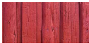
1 THIN STARTLING RED CEDAR PLANKS: EXTERIOR WALL
