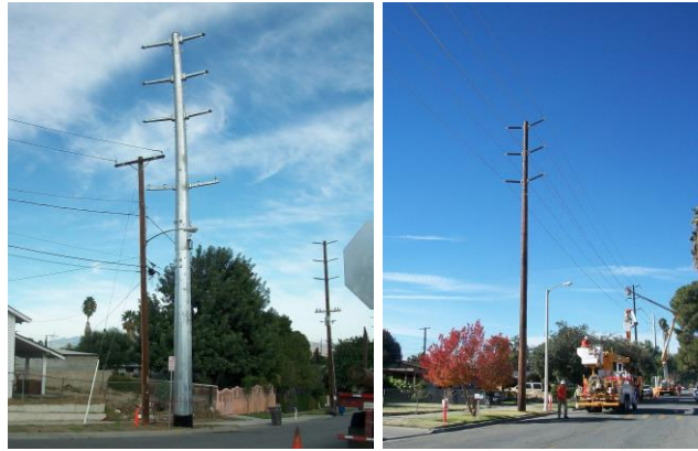
Typical 69kV overhead sub-transmission line work
