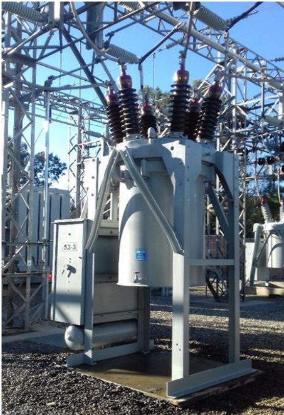
Typical Oil Circuit Breaker (Aged Unit)
