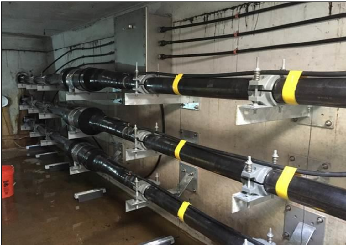
Typical 69kV underground cable installation work
