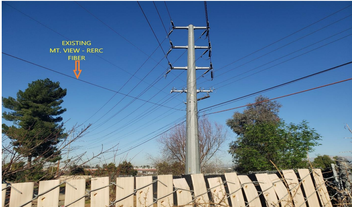
Existing fiber cable to be upgraded with new 144-strand fiber cable
