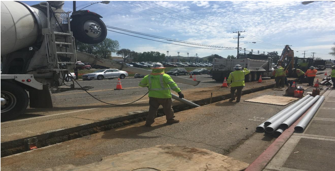
Typical trench and conduit installation
