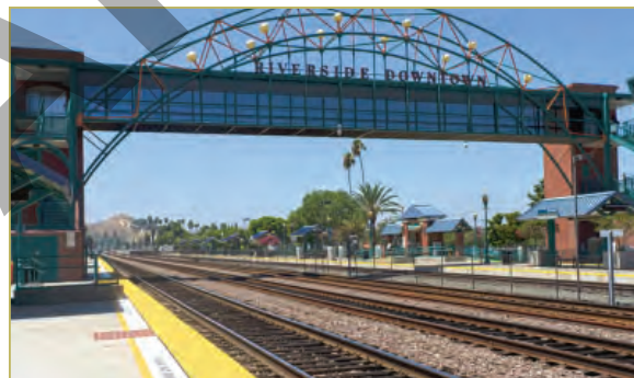
Riverside-Downtown Metrolink Station. Source: RCTC
