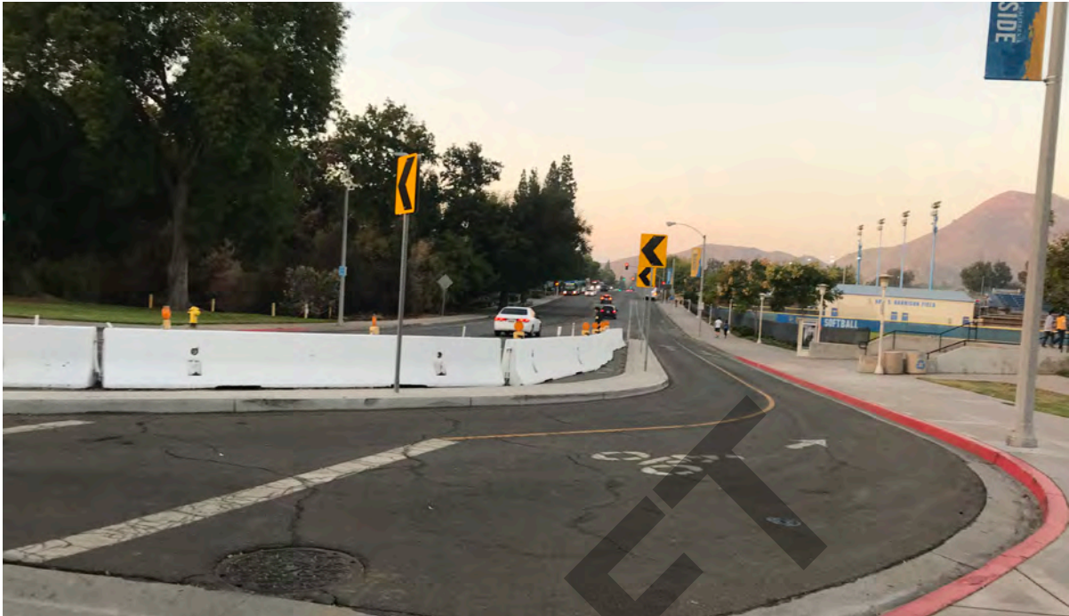
Photo Caption: Class IV Separated Bikeway along Canyon Crest Dr.
