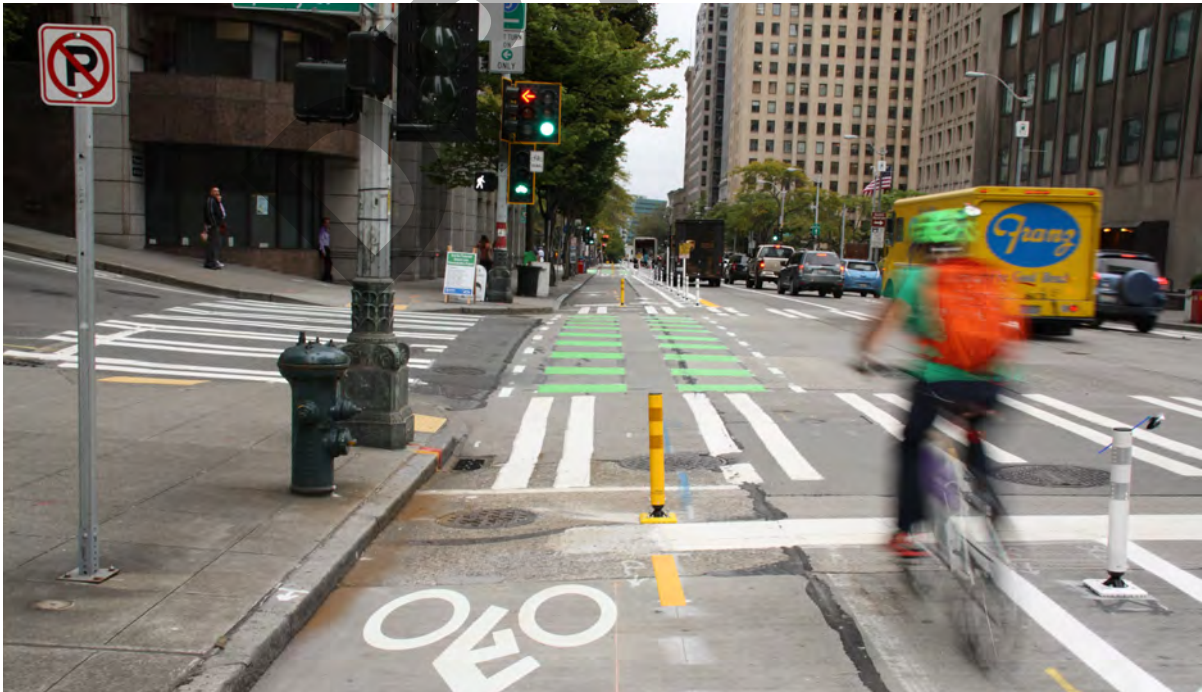
Photo Caption: Class IV Separated Bikeway in Seattle, WA.
