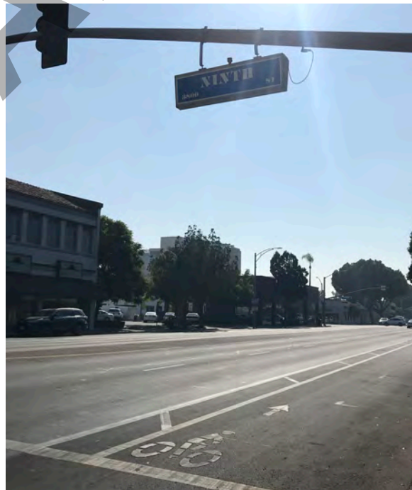
Photo Caption: Class II Bicycle Lane located on Market St.
