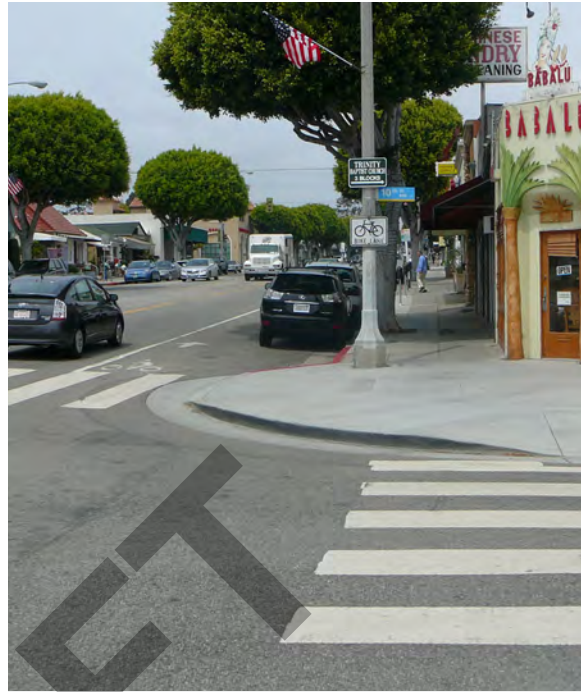
Photo Caption: Curb extension located in Santa Monica, CA.
