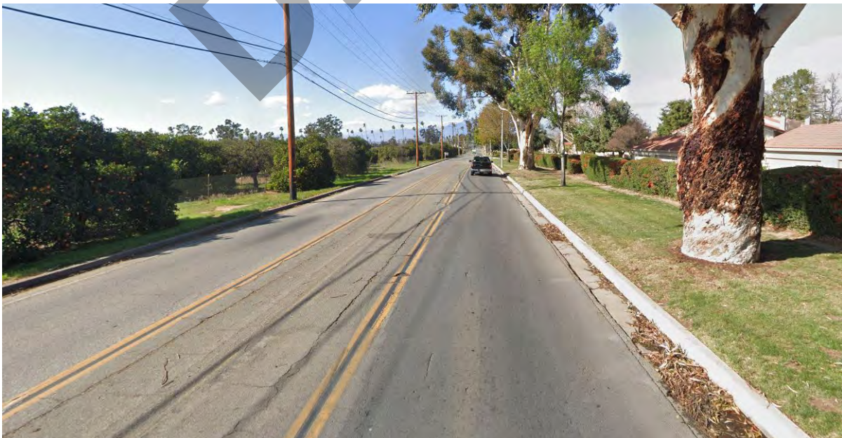
Photo Caption: Missing sidewalks along Washington St.
