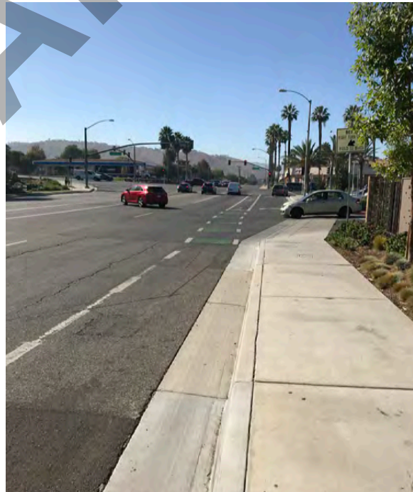
Photo Caption: Typical sidewalk condition along Indiana Ave.
