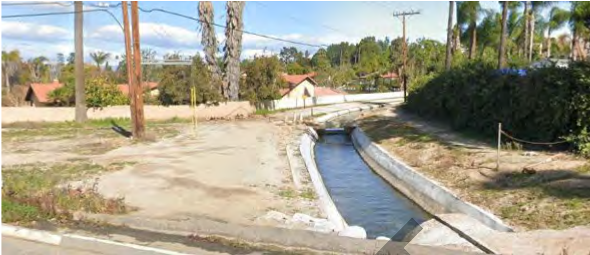
Photo Caption: Gage Canal crossing at Washington St
