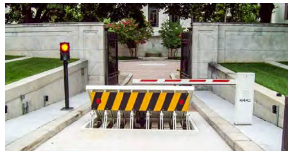
Examples of active barrier: surface plate shown above
