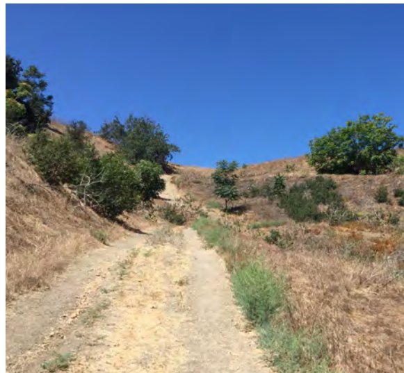
Long, straight sections of steep trail can lead to long-term erosion issues
