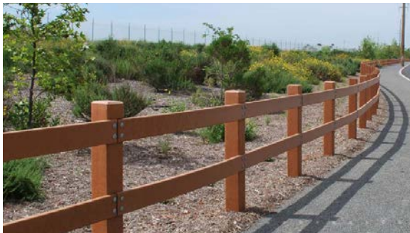
A 2-rail fence showing posts oriented toward the outside of the trail and rails facing towards the trail. Five Coves Wetlands, Anaheim, CA
