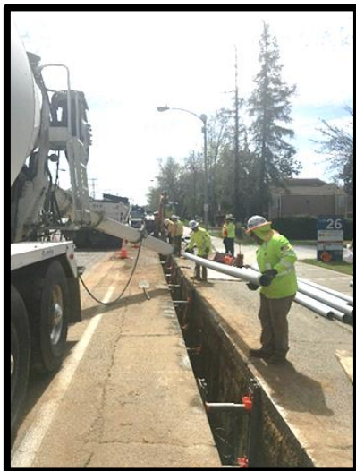
Typical Trench and Conduit Installations
