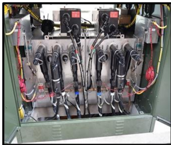
Typical Pad Mounted Switch W/ Protection
