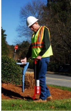
Typical underground facility locating process
