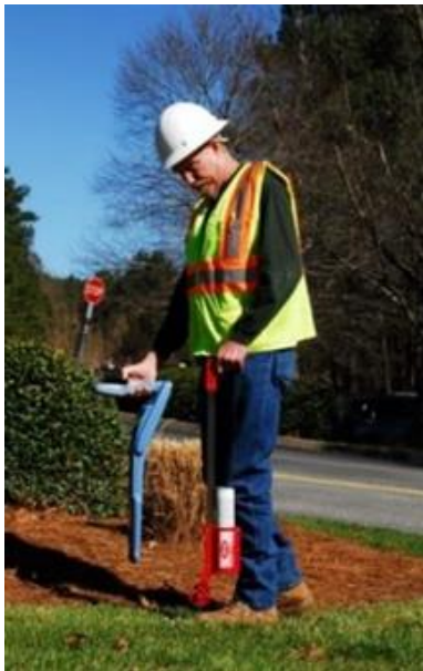
Typical underground facility locating
