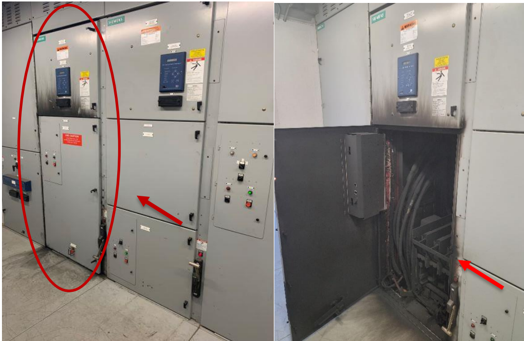
Figure 1 Photos of Failed Switchgear, August 28, 2020.
