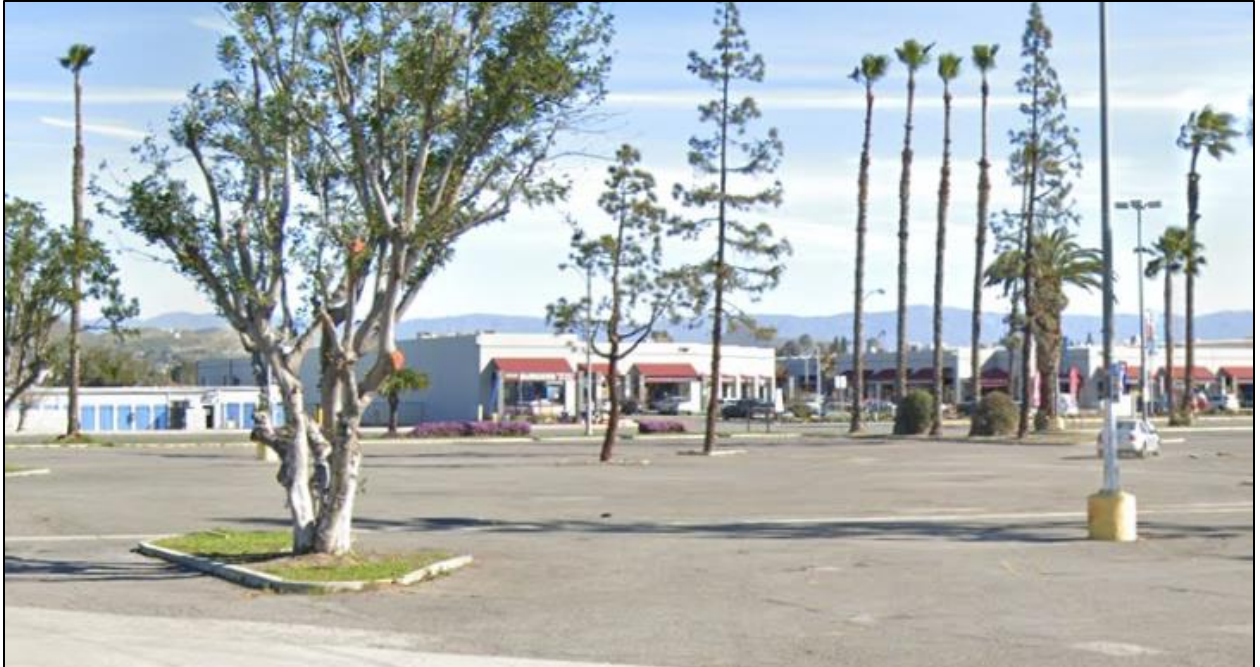
South Elevation (View from parking lot)
