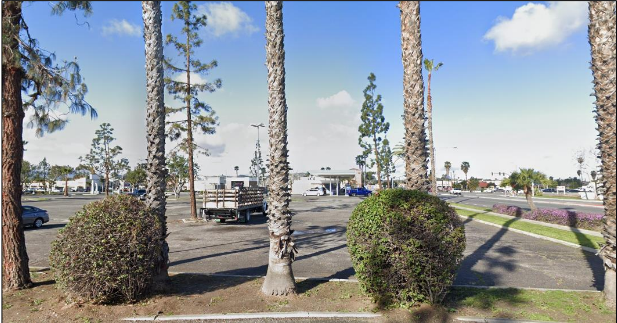
East Elevation (View from parking lot)
