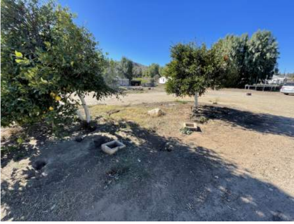
19. Potential leach field for septic on house at 6244 La Sierra Avenue
