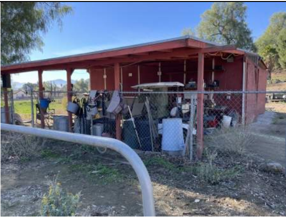
15. View of maintenance shed and overhang on central portion of Subject Property
