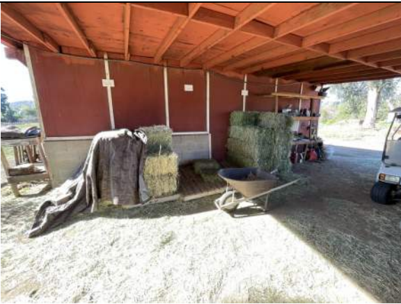
3. Bales of hay located underneath overhang on central portion of Subject Property
