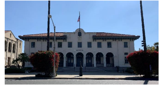
Maintaining 4 historic sites (7 sites total)
