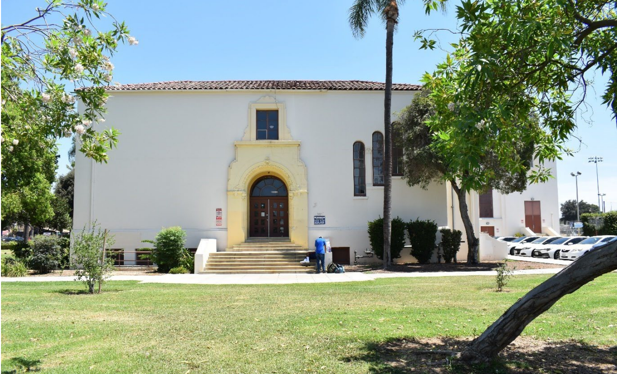
Photograph 8. West Elevation, Including Formal Entrance, Facing East
