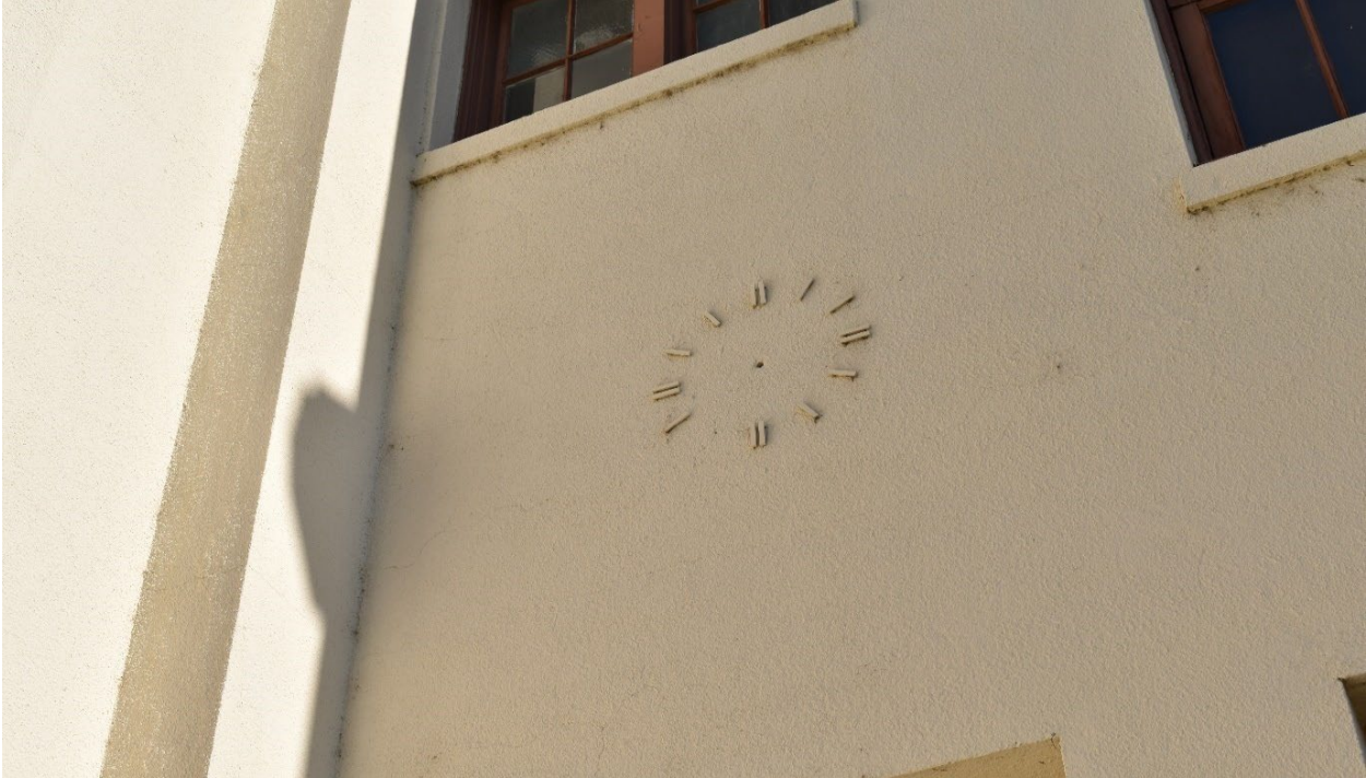
Photograph 9. Integrated Clock Above South Elevation Entrance
