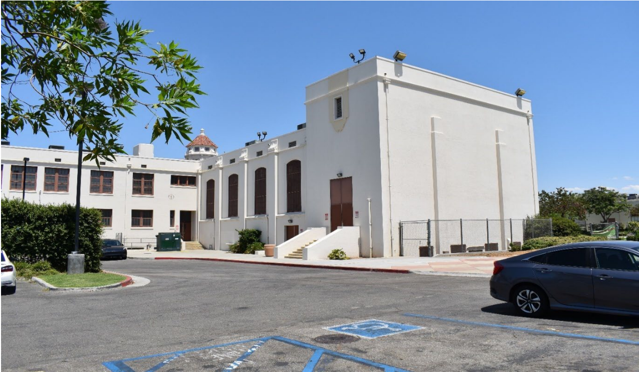
Photograph 10. Exterior of Auditorium, South and West Elevations, Facing Northeast
