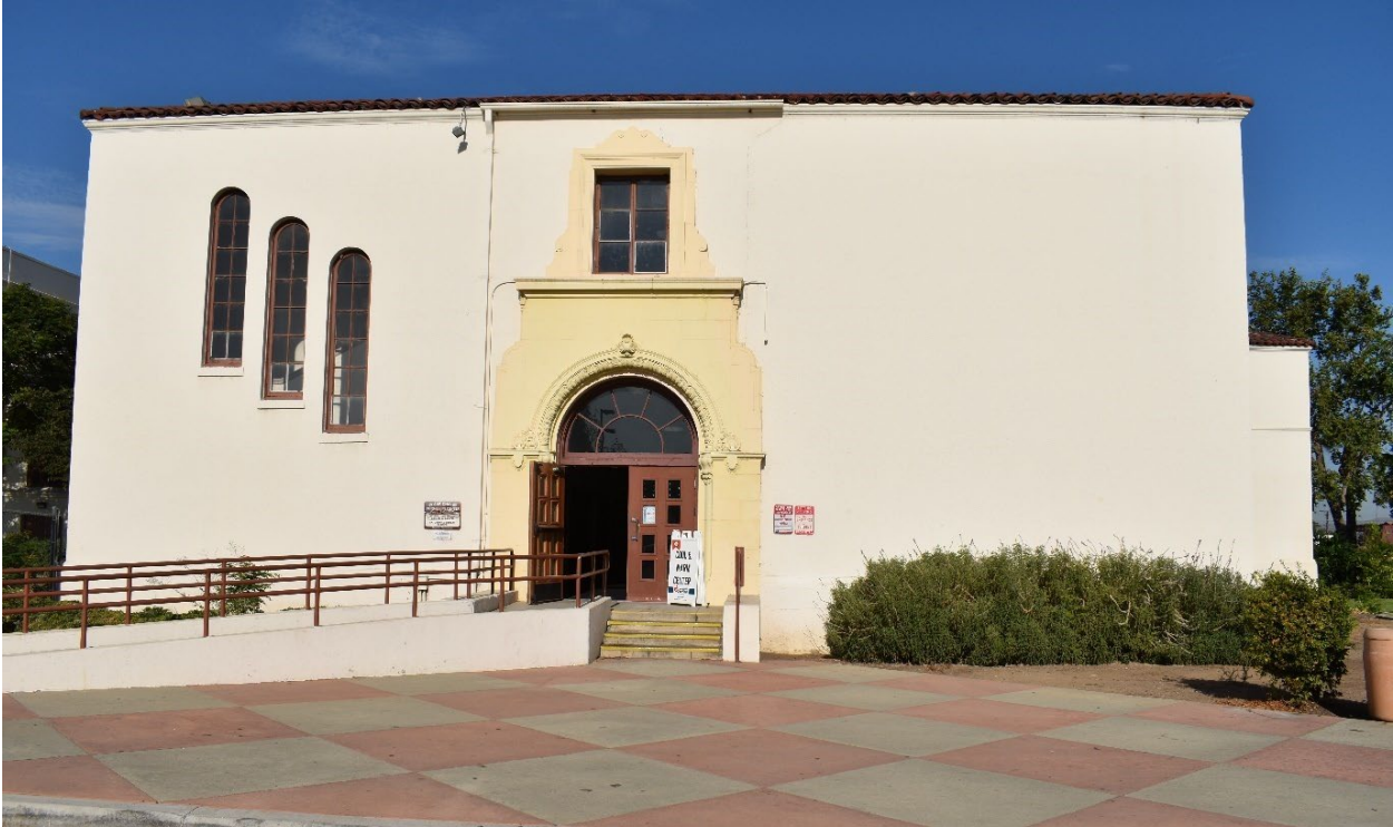
Photograph 7. East Elevation (Partial), Featuring Formal Entrance and Stepped Stairwell Lights, Facing West
