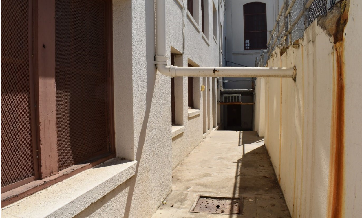
Photograph 11. Representative View of Sub-Grade Access Area, Facing East
