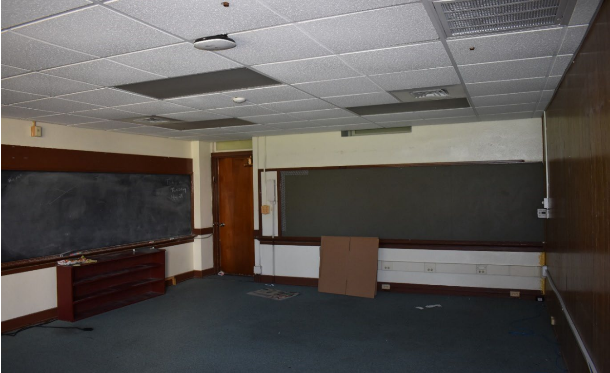
Photograph 16. Overview of Representative Classroom with Non-historic Partition at Left of Frame
