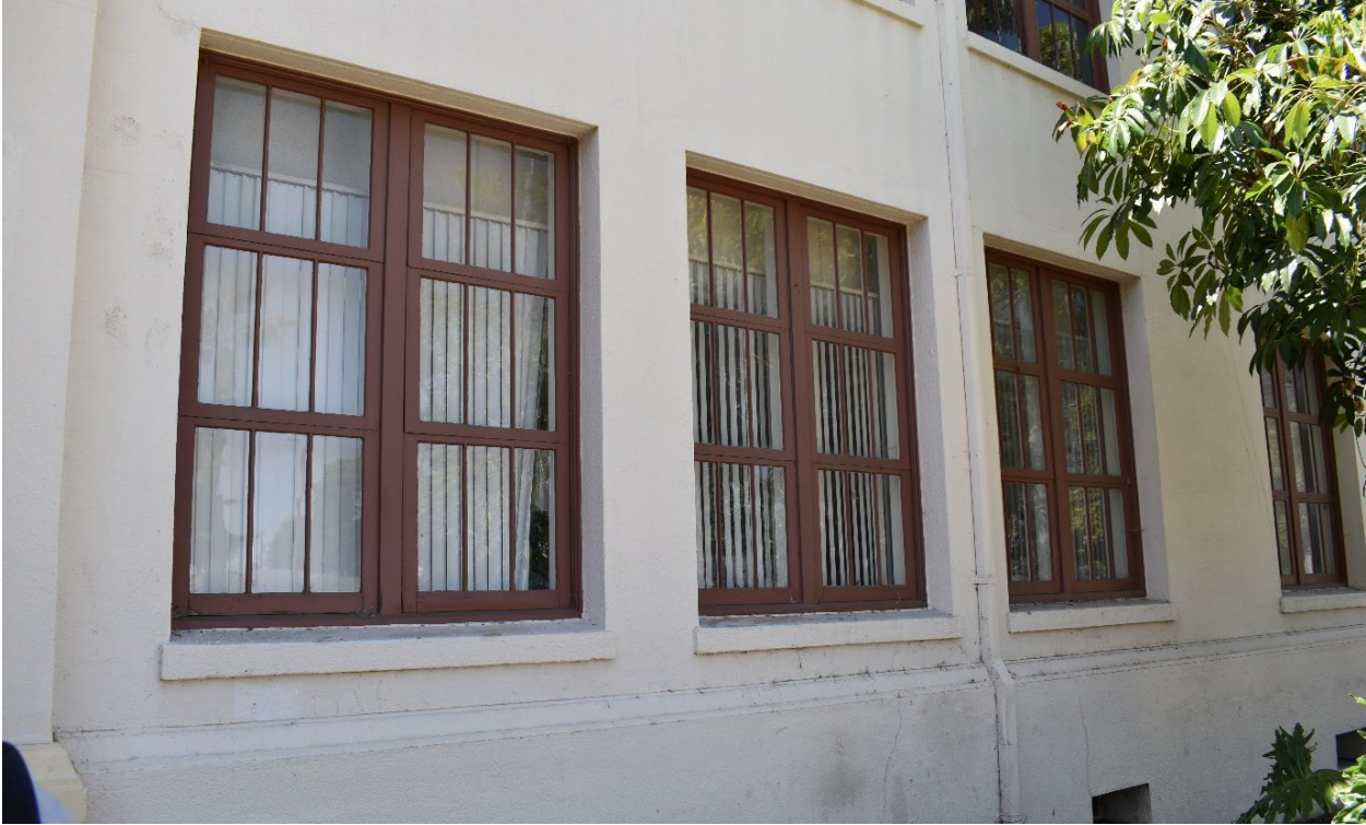
Photograph 4. Typical Wood-Sash Awning Window on North Elevation
