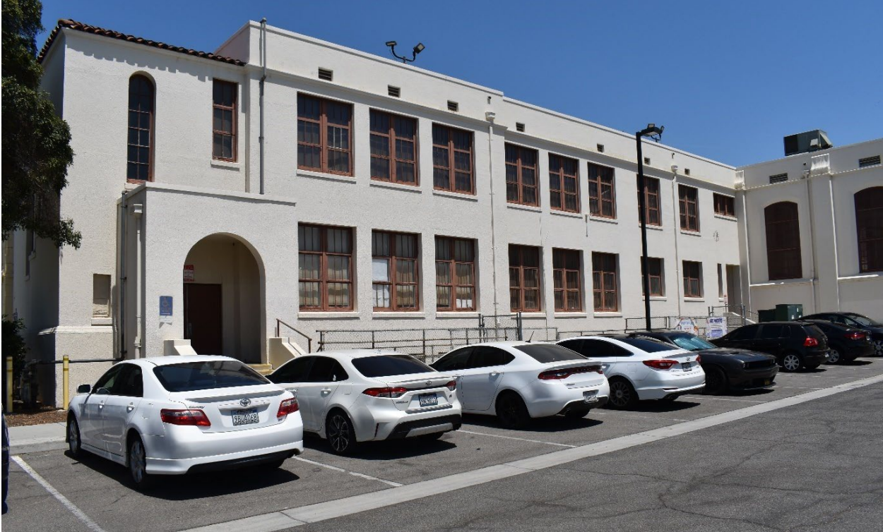
Photograph 5. South Elevation, Featuring Typical Fenestration, Facing Northeast
