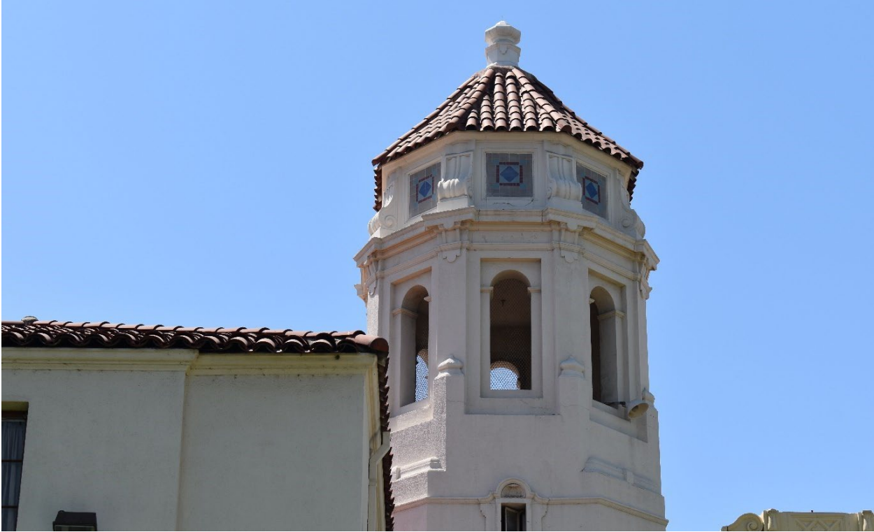
Photograph 3. Upper End of Tower Feature, Facing South
