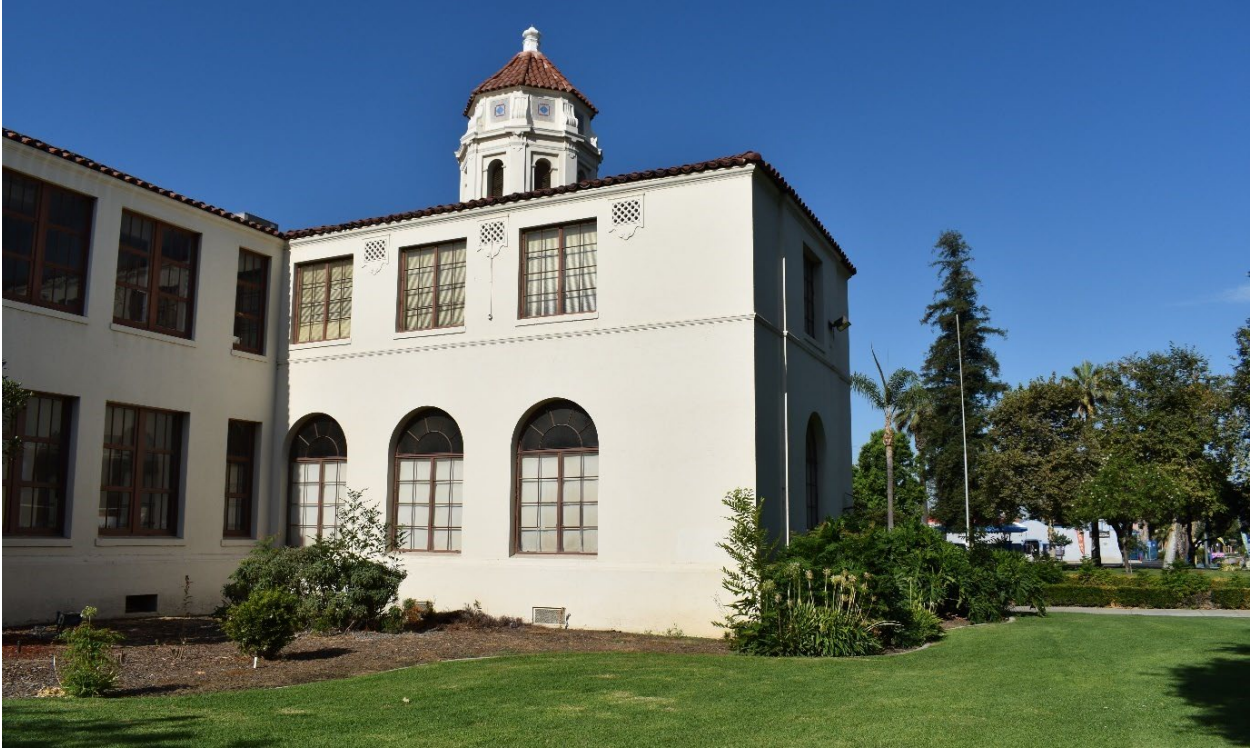
Photograph 6. North Ell, Displaying Typical Fenestration, Facing Southwest
