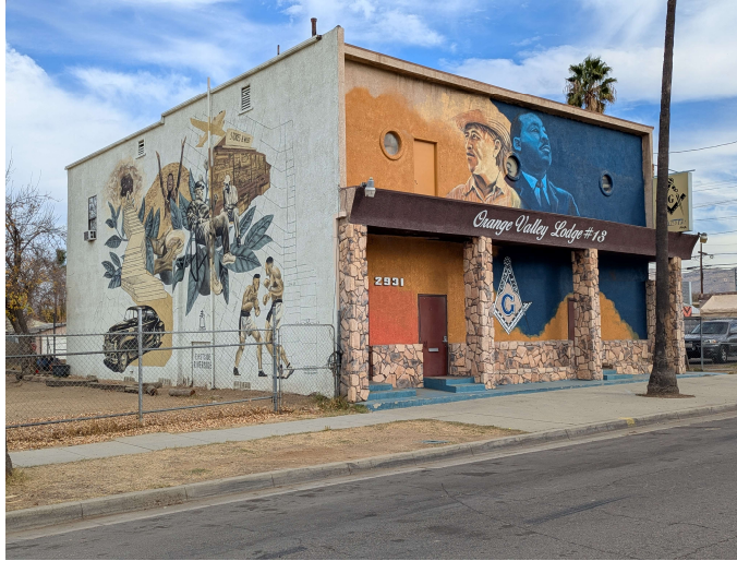
Current building façade
