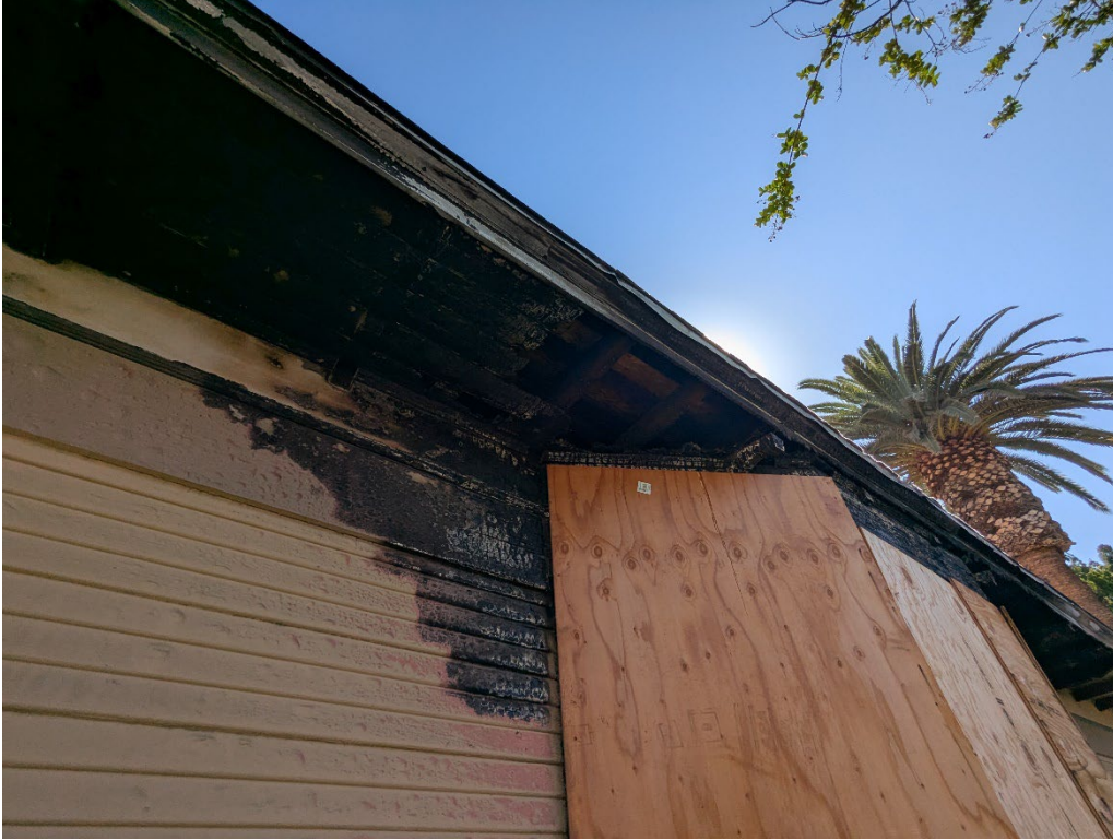
Figure 9 - South side fire damage
