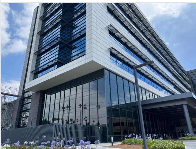
24. East Adjoining Property
