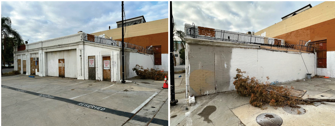
Restroom Addition (by 1952) and Later Addition (date unknown) to Service Station
