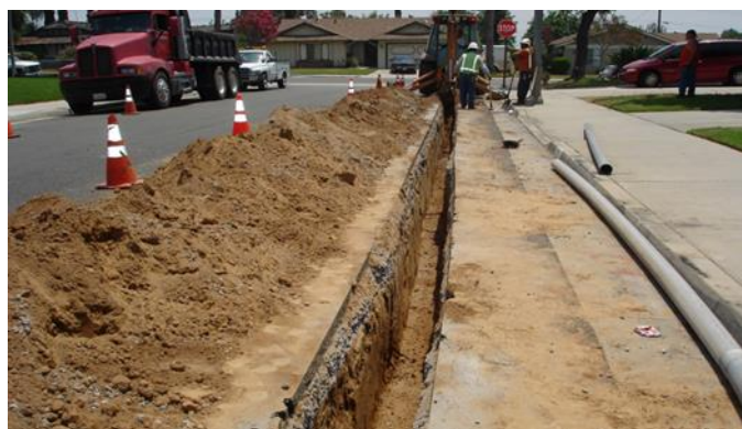
New trench and conduit installations
