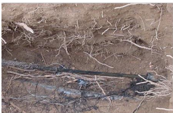
Aged Infrastructure: Cable-in-Conduit System
