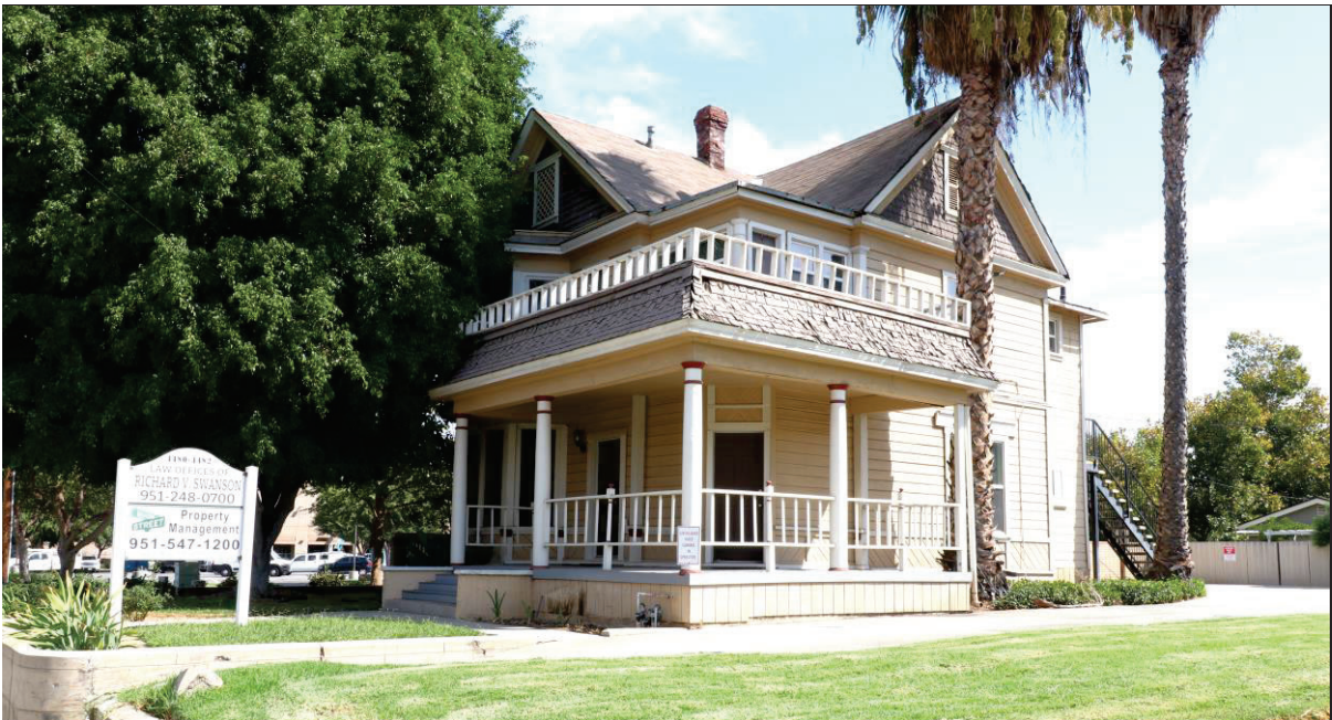
Photo 13. Offices at 4480–4482 Main Street, view northeast (10/7/24).
