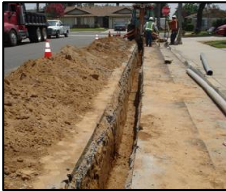
Trench and Conduit Installation
