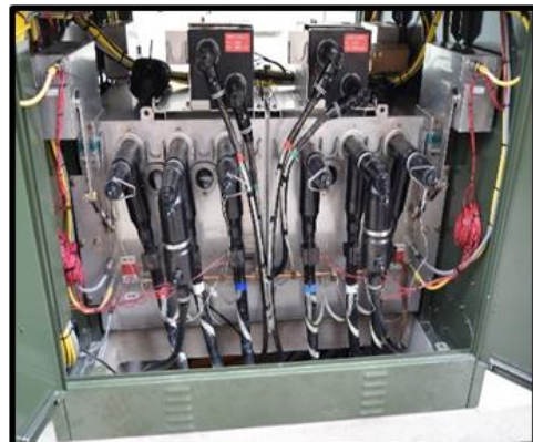
Typical Padmounted Switch W/ Protection
