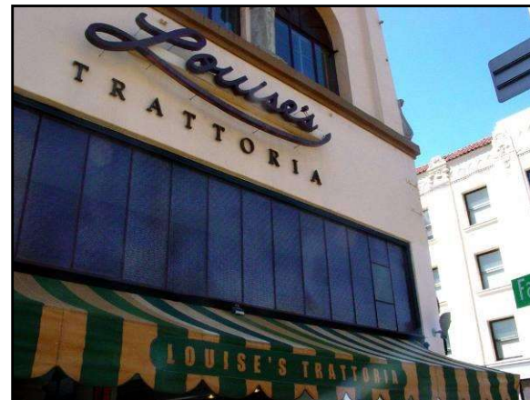
Encouraged: Placement of wall-mounted sign directly above the storefront respects and accentuates the building's architecture.
