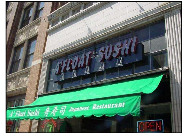
Discouraged: Wall-mounted sign covers transom windows and would be better located above.
