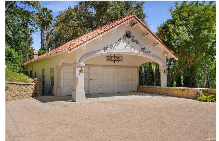
Detached Garage/Caretakers Unit
