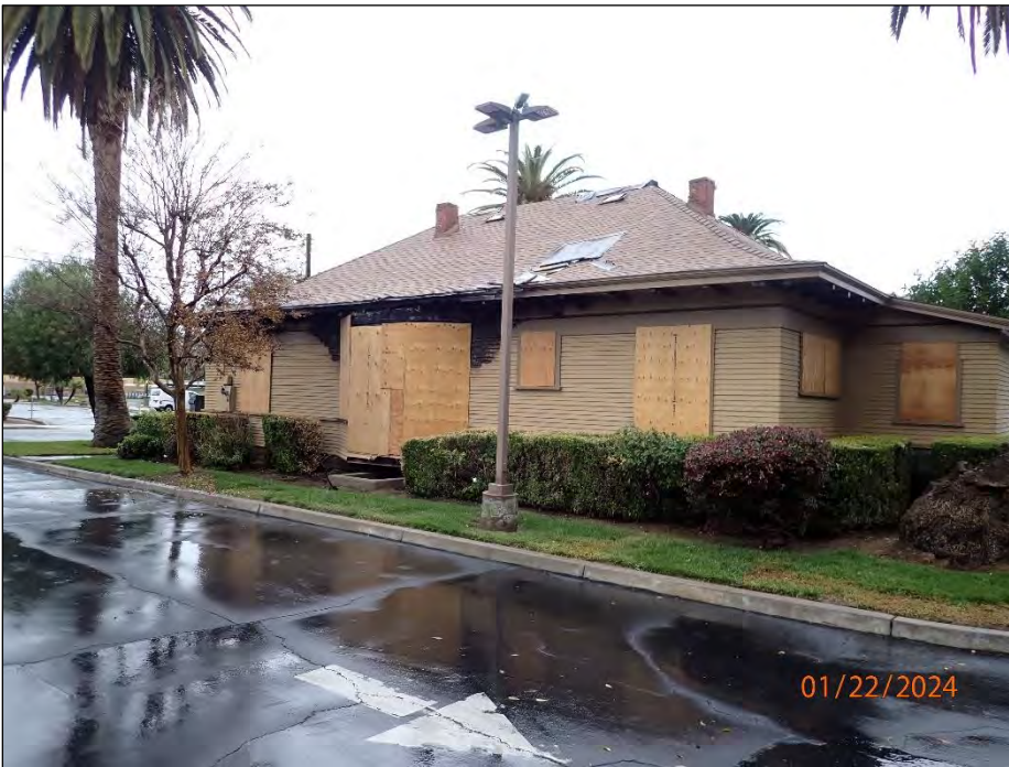
2. View of the east and south exteriors of the building from the parking lot. Wall/window openings had been boarded with plywood subsequent to the reported fire event.
