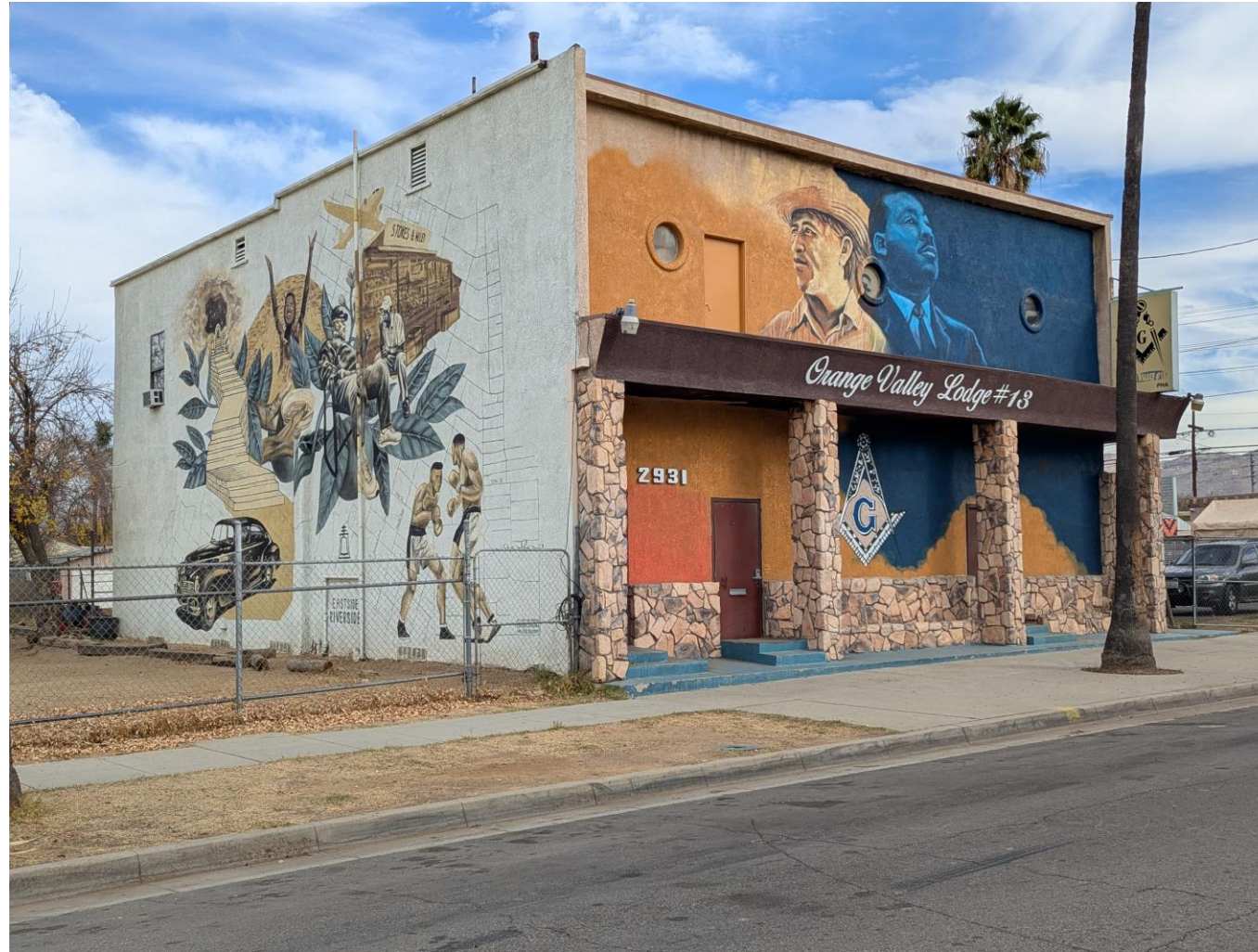
Current building façade
