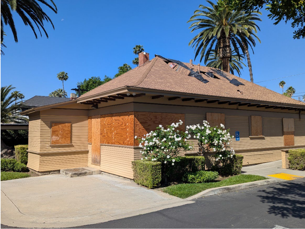
Figure 5 - East and north elevation, view looking southwest
