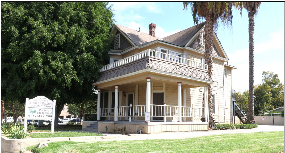
Photo 13. Offices at 4480–4482 Main Street, view northeast (10/7/24).
