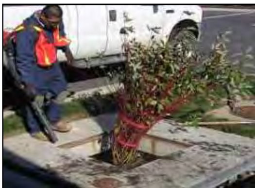
5. Clean area around Filterra
