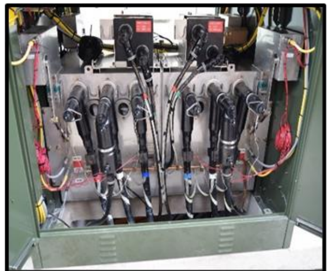
Typical Pad Mounted Switch With Protection
