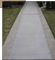
TROWELED FINISH BANDING AT PAVING EDGE
